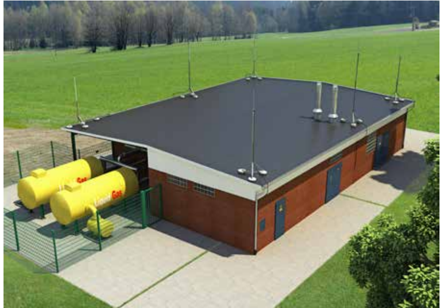
Abb. 6: isCon ® Pro+ conductor on air-termination rod in Ex area
