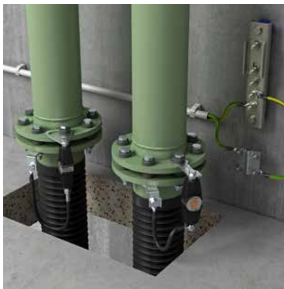
Abb. 4: Spark gap mounted on insulating sections
